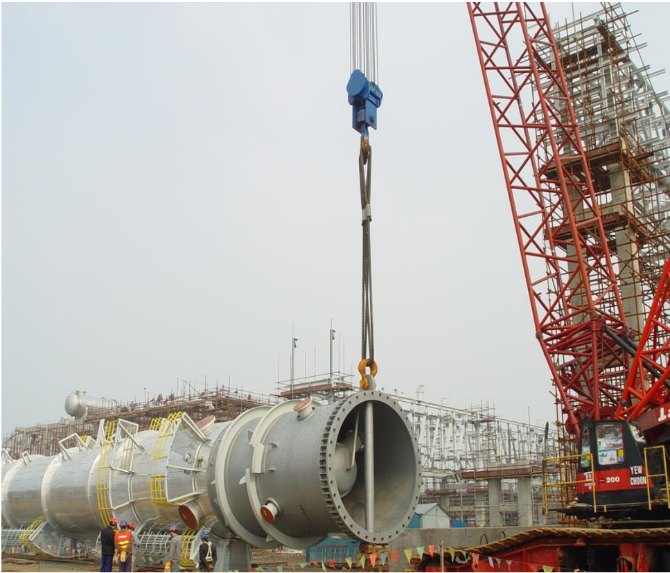
The next photo is just a close up of the first one. Note that this basering has type 2 chairs, ie, it has a top ring and a bottom basering. Also notice that the tail lug is located between the anchor bolt holes.
