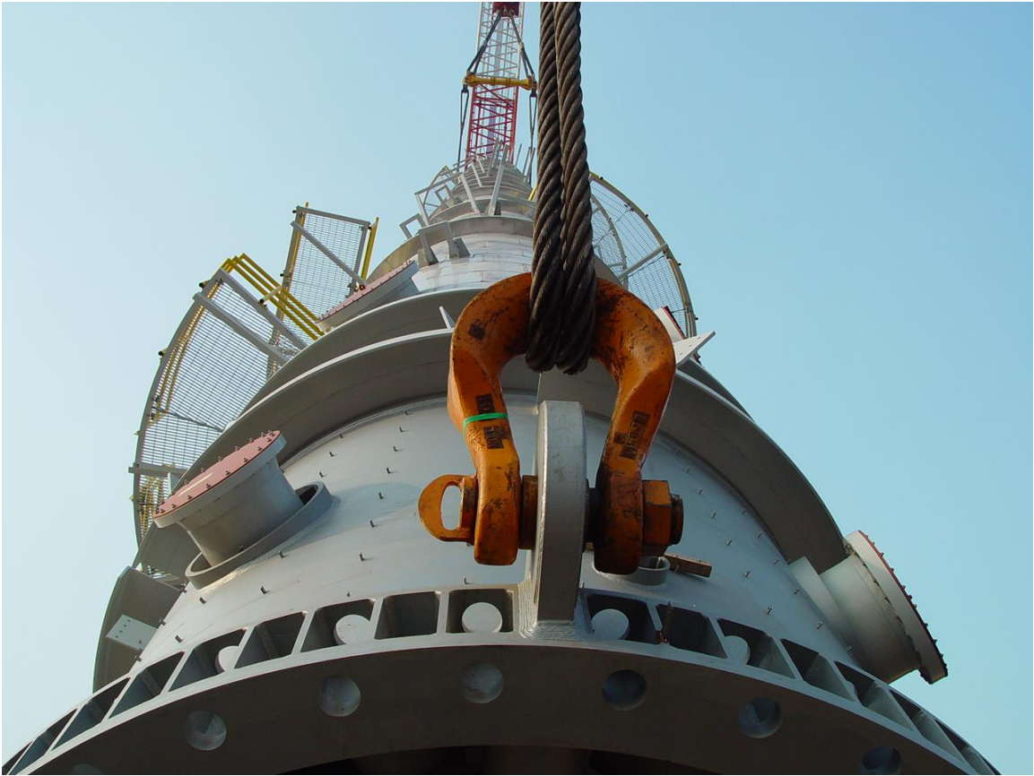
The next photo is just a close up of the first one. Note that this basering has type 2 chairs, ie, it has a top ring and a bottom basering. Also notice that the tail lug is located between the anchor bolt holes.
